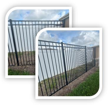
A few metal posts were found damaged along the fence, and these have been replaced.
