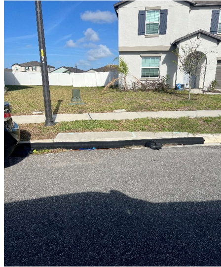
Stormwater Inlet Blockage (typ.)
