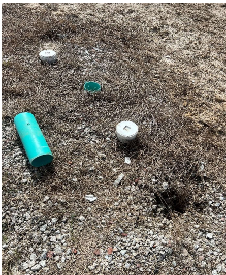
Damaged Cleanout
