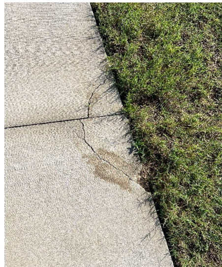
Cracked Sidewalk
