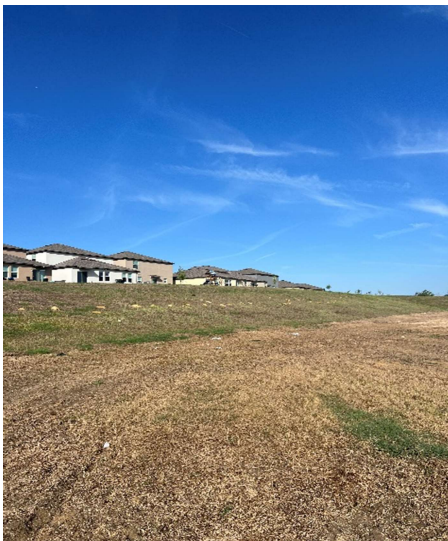
Debris/Trash in Pond (typ.)
